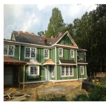
Energy House Five is moving forward quickly. With the framing being finished, siding is about to start and the insulation is being installed, some exciting things are to be reported about how this project is different from most of the homes being built today. This ENERGY STAR home is a perfect example of advanced framing standards that are helping to make this project one of the most energy efficient homes in the Alexandria community.
