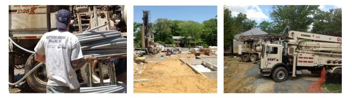
Energy House Geothermal – Four tons of heating and cooling has been drilled into the driveway area of the site. Two Closed Loop Wells
