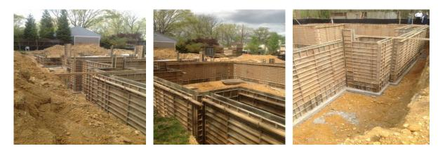
The actual pouring of the concrete on Energy House Five was done by Federal Contracting with a concrete pump truck rather than just being poured by a cement truck. This ensured that the pour was perfect with the proper amount of compacted concrete reaching corners of the foundation so no fissures or cracks occurred once the forms were stripped and removed. It was done excellently by Federal Contracting and their subcontractors.
