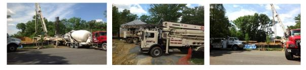
Once the concrete pour is complete, it is given a few days to set and harden and then the forms are stripped and we have foundation walls. Another wall check is done by the engineering company to make sure all is in its exact location and the next step is to pour the concrete slab floor.
