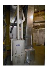
With a variable speed furnace, heat pump and programmable thermostats this is one of the most efficient HVAC systems ve can install.
